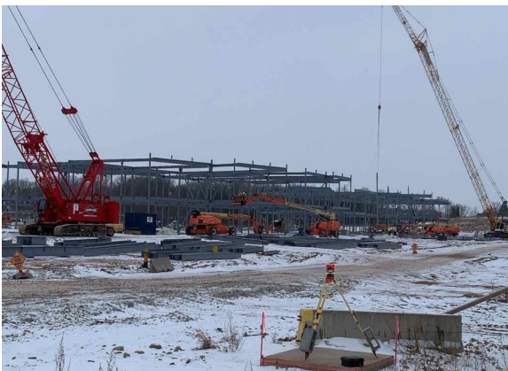
Entire north side of the building structural steel (02/24/2022)
