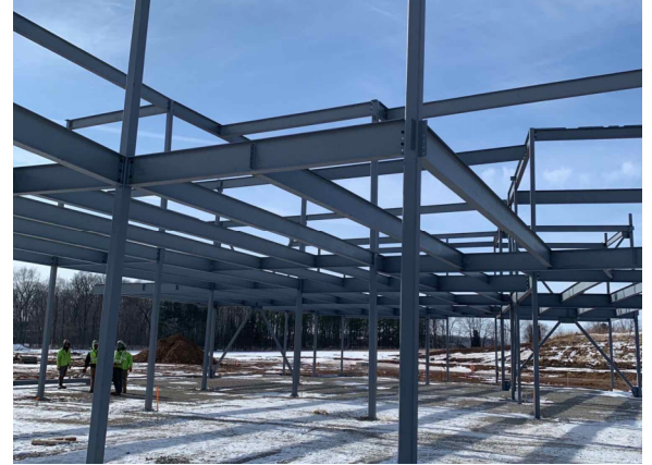
Structural steel going up in West classroom wing (02/08/2022)
