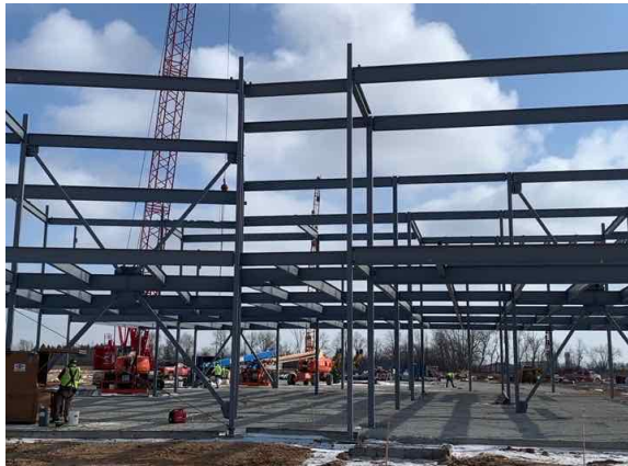
Structural steel in East classroom wings (02/14/2022)
