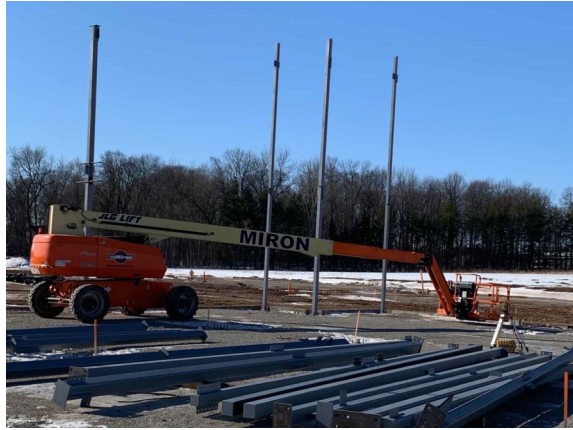
First day of structural steel in West classroom wing (02/03/2022)
