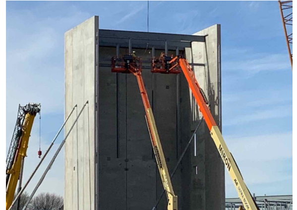
Auditorium precast walls get braced with structural steel at the top (02/28/2022)
