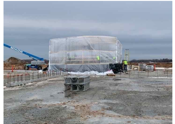
Heated masonry enclosure next to future weight room (02/16/2022)
